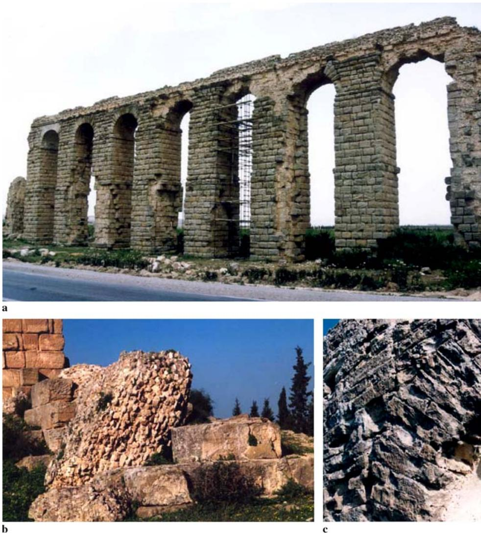
**FIGURE 3** Aqueduct of Carthage: (a) Roman arches in risk of dismantling being subjected to consolidation works; (b) fallen-down blocks of opus caementitium and original sandstone ashlars (c) detail of ashlar blocks displaying stone alteration by alveolization
